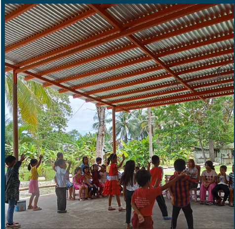
New roof at Kimaya Elementary
