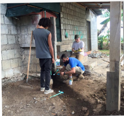
PREPARING FOR A NEW LAUNDRY AREA
